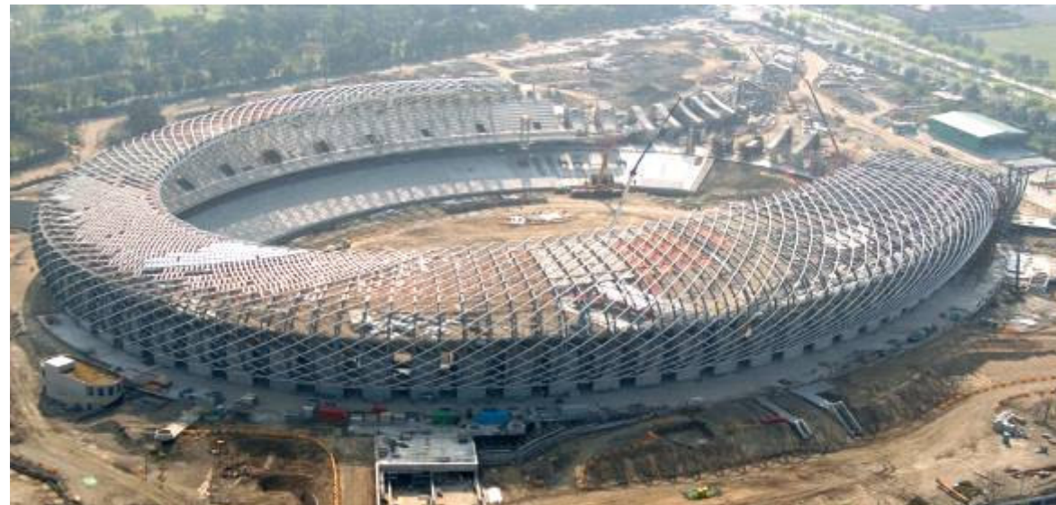
Kaohsiung Arena's 1MW BIPV System (w/ Delta's Inverters & DeSolar's Cells)
